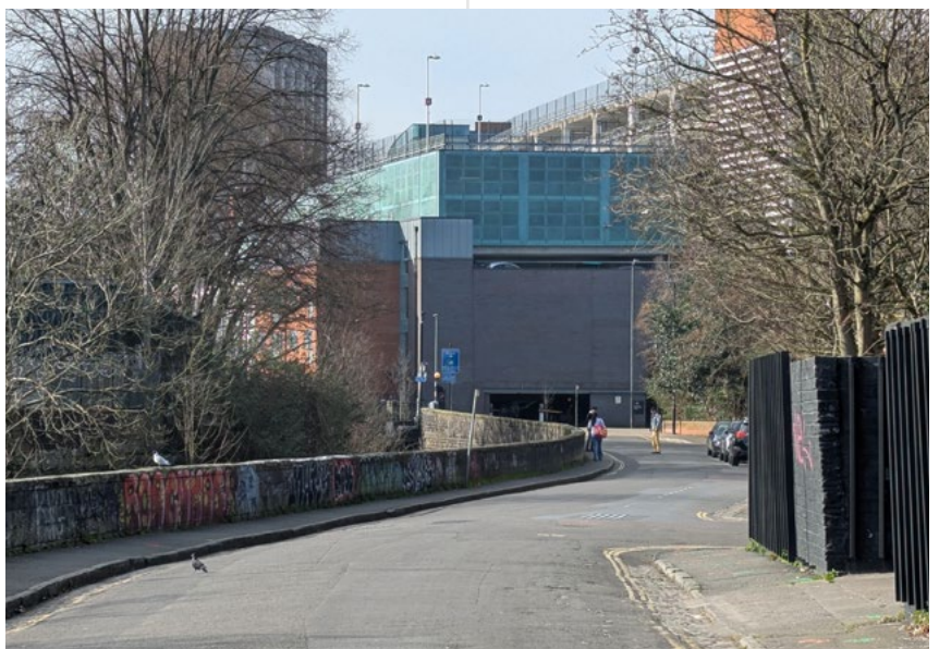
Wellington Road looking towards Wade Street
