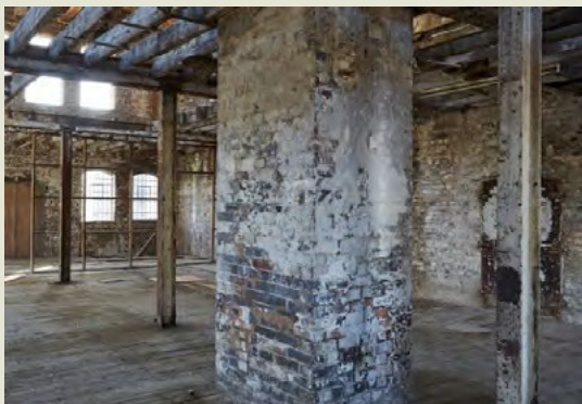
Example: Grand Union, Junction Works, Digbeth, Birmingham
